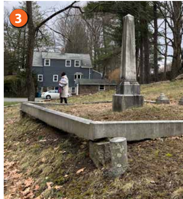
Eroded soil exposing coping foundations
