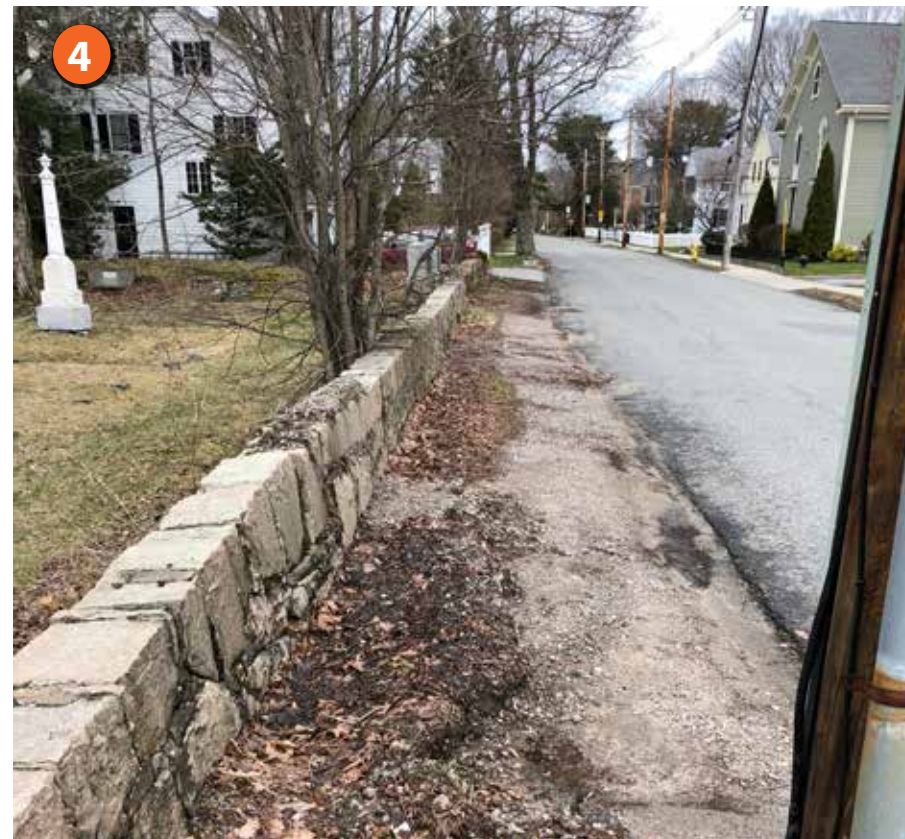
Failing mortar at stone wall, volunteer trees impact
