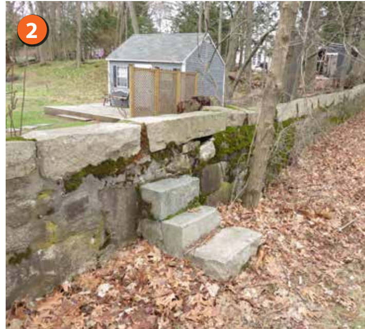
Tree impact to wall; broken wall with failing mortar
